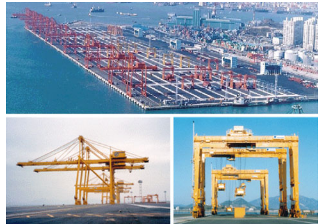
Fig. 1 – Gantry crane auto-steering system based on GPS carrier phase measurements.
