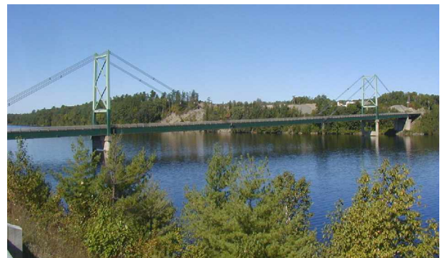
FIGURA 1 – Hawkshaw Cable-stayed Bridge in New Brunswick, Canada
